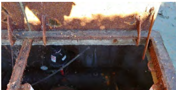
Photo 1 Rusted Underside of Access Hatch
