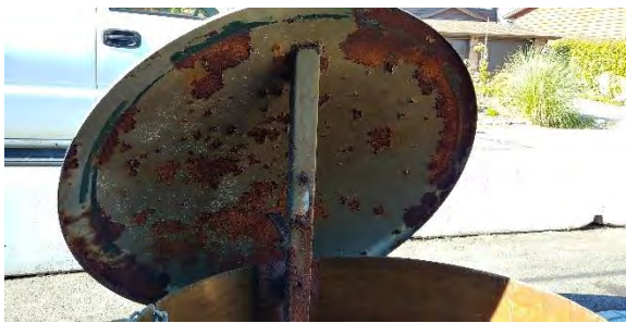
Photo 1 Underside of the Steel Access Hatch
