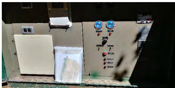
Photo 1 Minor rust on Electrical Kiosk
