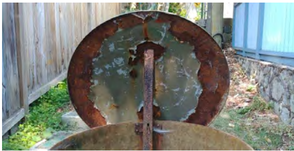
Photo 1 Rusted Underside of Access Hatch
