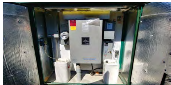
Photo 2 Chemicals and Dosing Pump
